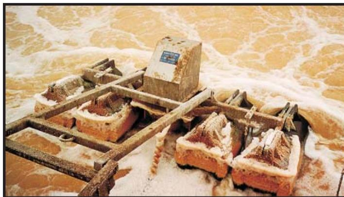
**This AquaTec decanter is shown operating in sub-zero conditions in an AquaTec SBR system designed for treatment of high strength dairy waste. It operates flawlessly and constantly produces high quality effluent.**
